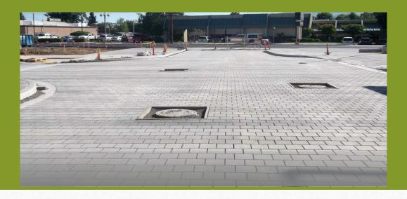
Mostly used in the form of porous pavers similar to cobblestones, these pavers slow the flow of water and allow it to soak directly into the ground as it would in a natural environment.
